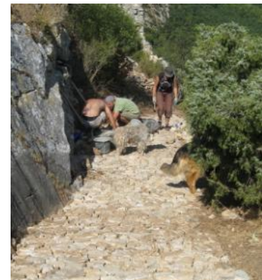
Restoring the path
